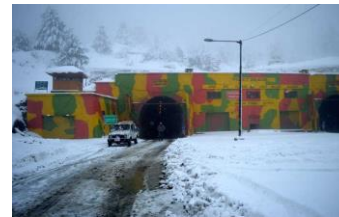
Jawahar Tunnel, J&K
