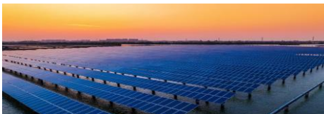
DVC 35 MW Solar Project
