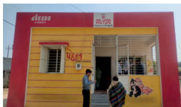
Construction and renovation of Anganwadi - Halol
