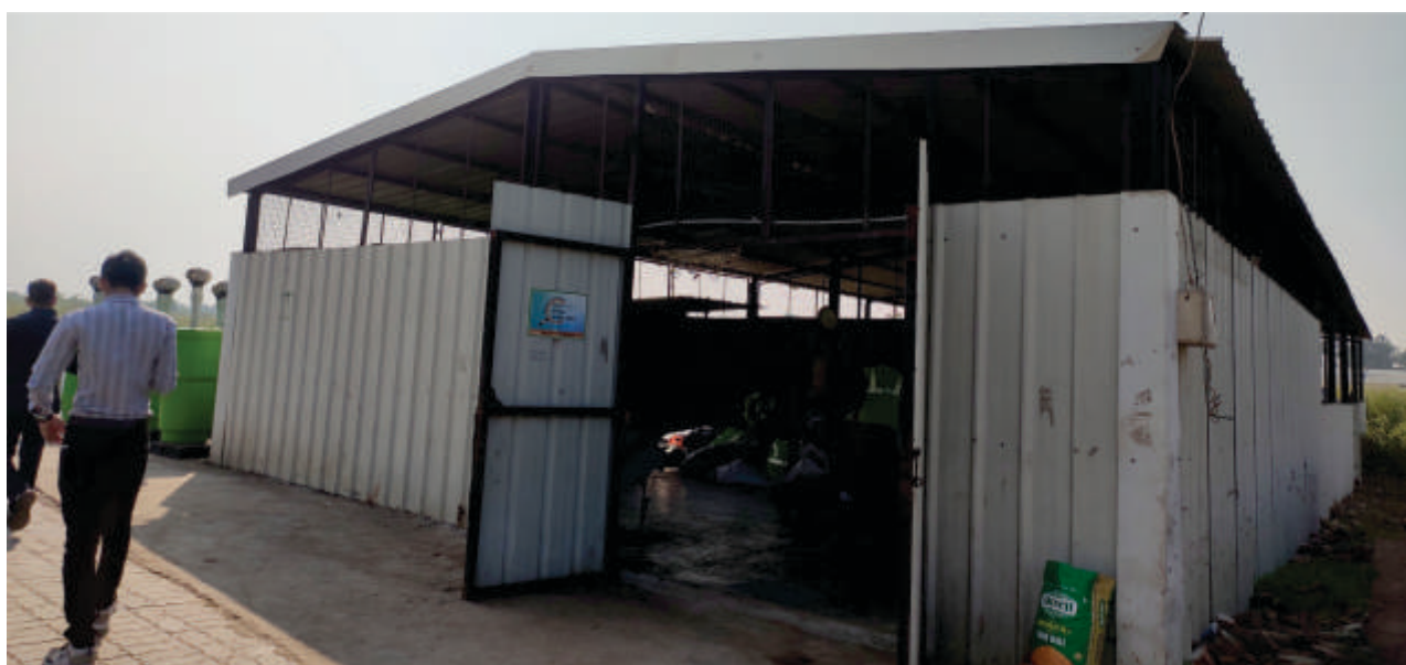
Waste Collection Shed - Halol
