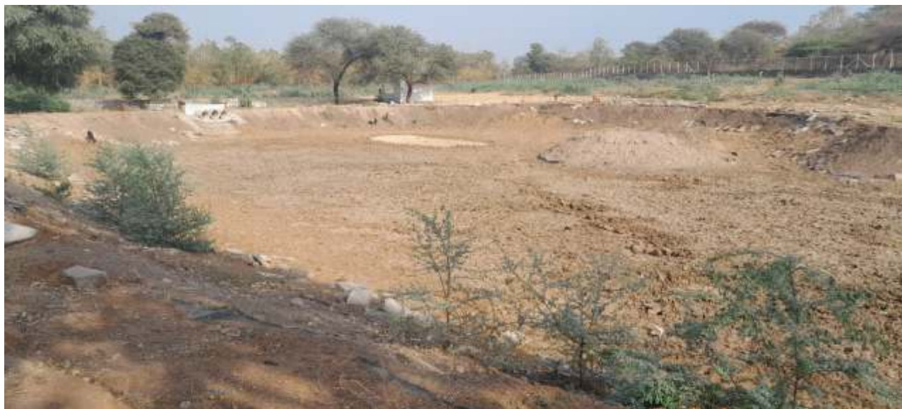
Pond deepening at forest restoration site and system of cement pipelines – Jepura
