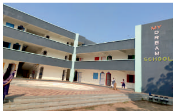
Construction of School - Halol
