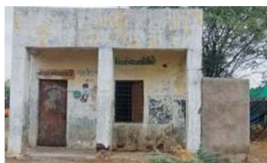
Above Photos of Previous Infrastructure Anganwadi centres - Halol
