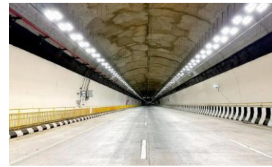
Kasara Ghat Tunnel
